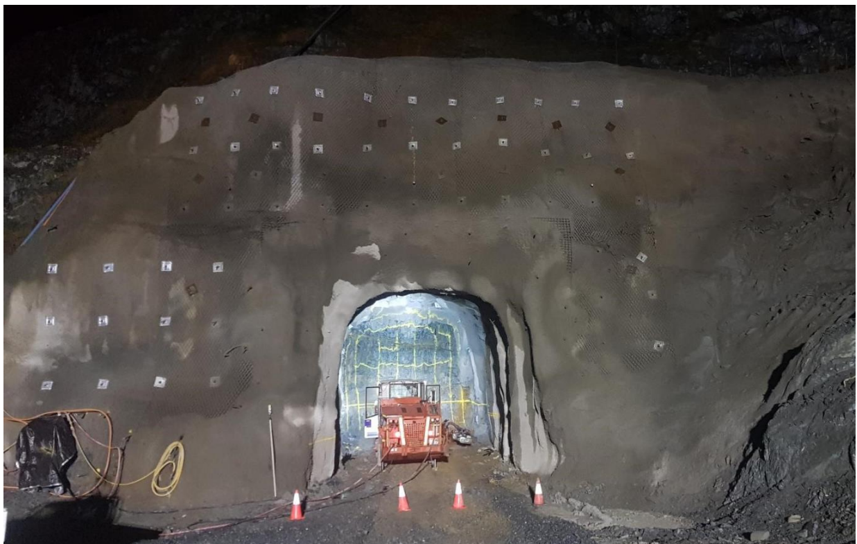
Figure 2 – Portal complete and decline progresses.
