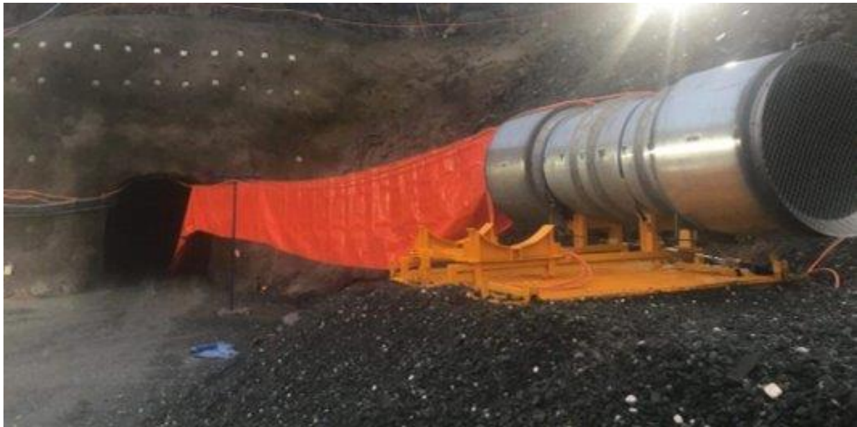
Figure 2 – new Fan and Ventilation installation
