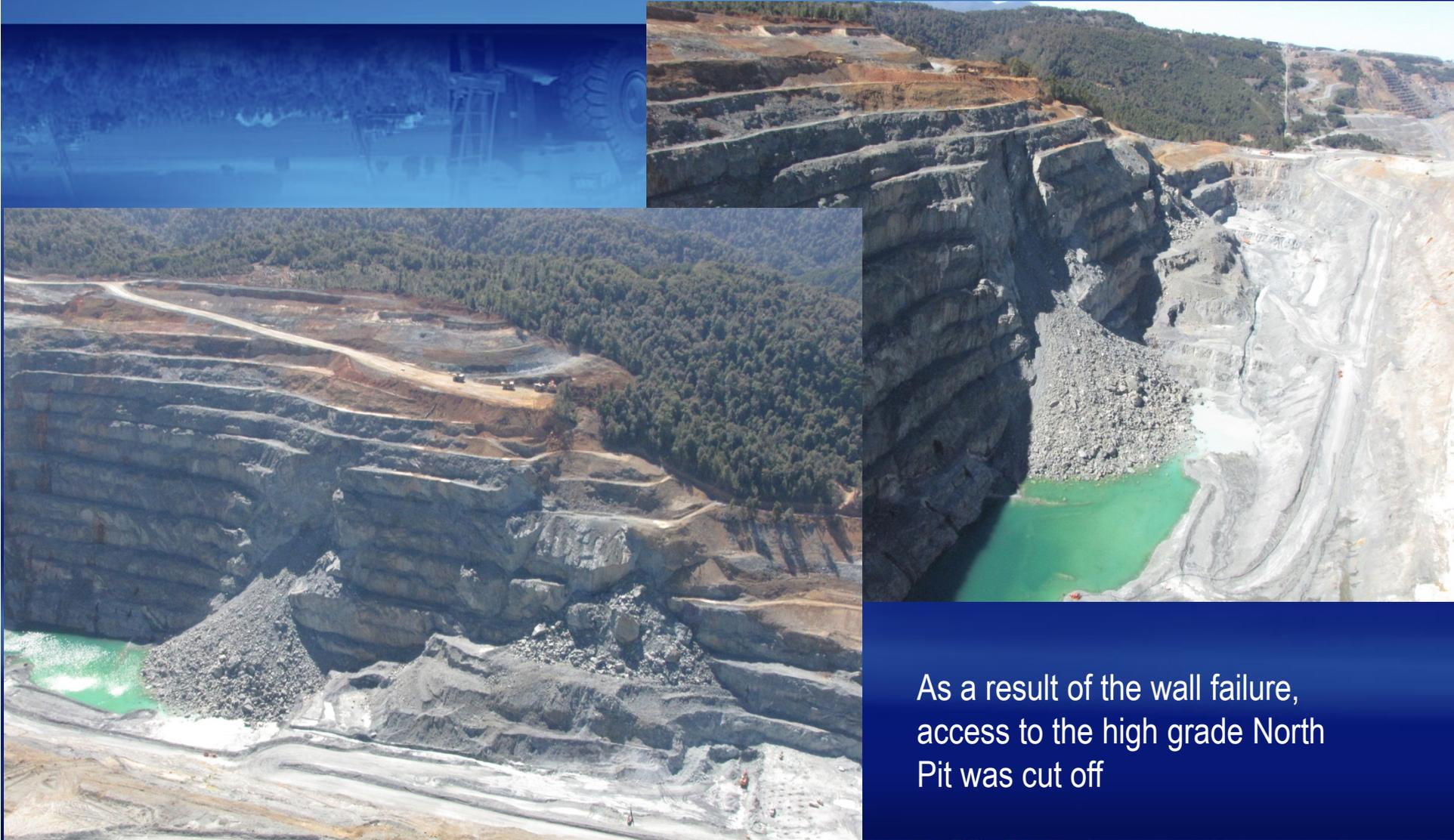
As a result of the wall failure, access to the high grade North Pit was cut off
